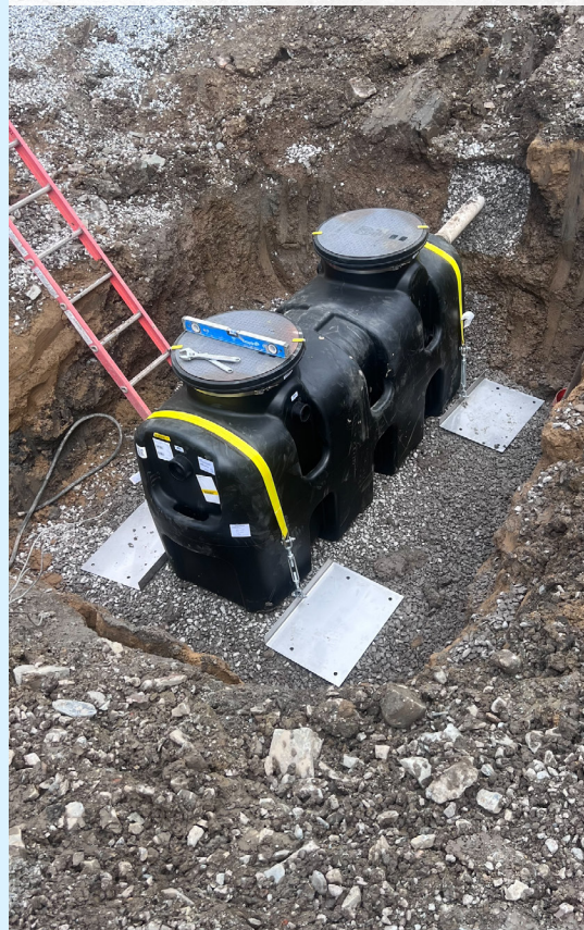
OS-350 | PARKING GARAGE
